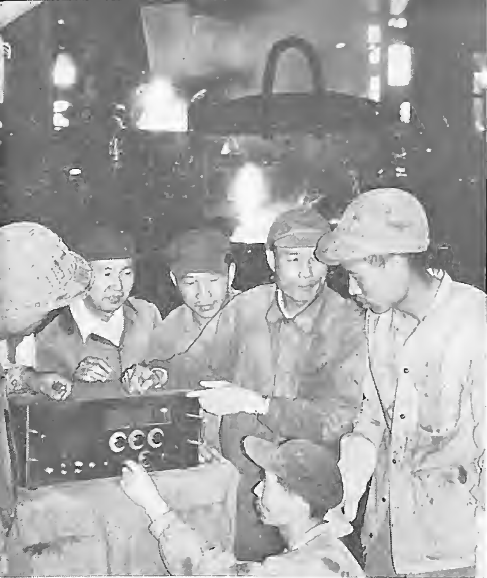
This electronic scale developed by the Shanghai No. 1 Iron and Steel Plant accurately controls the amount of iron poured into a ladle.
